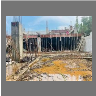
Commercial Construction Service
